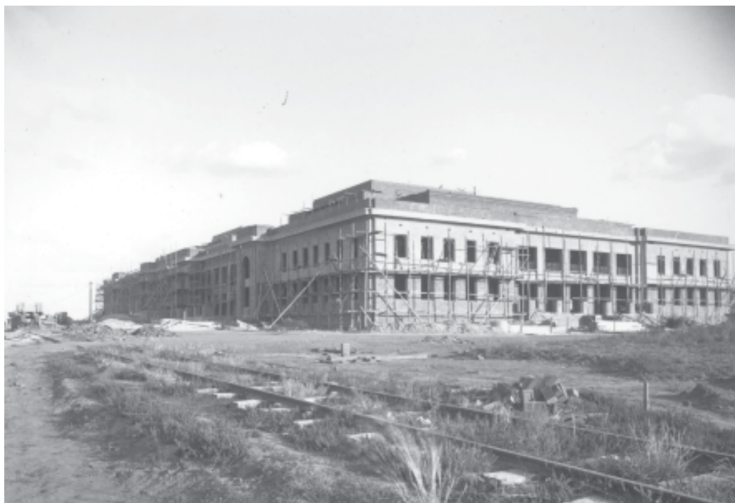
This view of Parliament House from the north west shows the tramway laid to transport bricks to the site direct from the Yarralumla brickworks.
