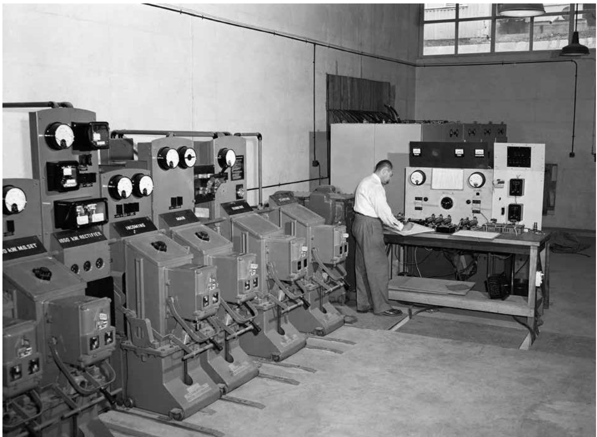
The switch-room unit, which served the 10 million volt proton synchrotron installation at the Australian National University, Canberra, 1955. Photographer: W Pedersen.
