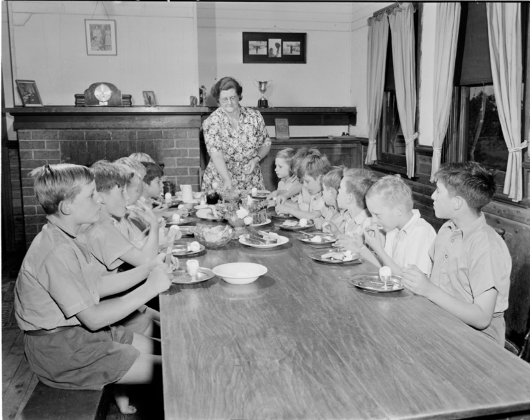
Breakfast at the Fairbridge Farm School at Molong, NSW, 1954. NAA: A1200, L17162
